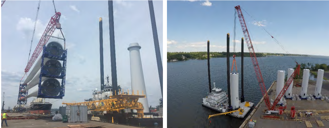
Photos of blade and tower loading operations at ProvPort that were managed by WTS
